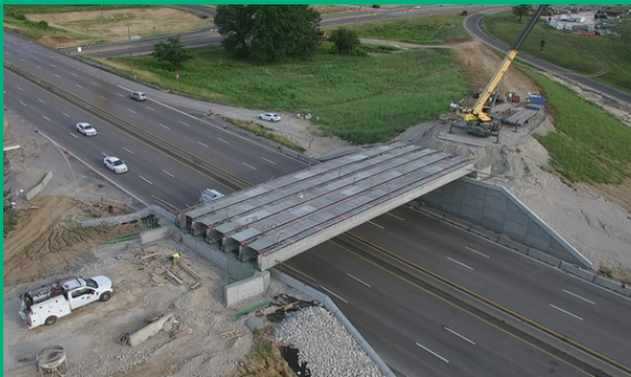
Route 367 Flyover Ramp
